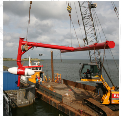
T100 TURBINE BEING INSTALLED
